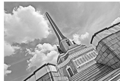
The Elevated Radial Platforms
